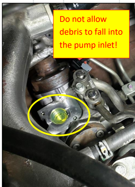
Figure 9: FCA Removed (no debris)
