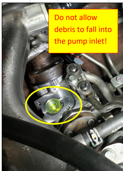
Figure 9: FCA Removed (no debris)
